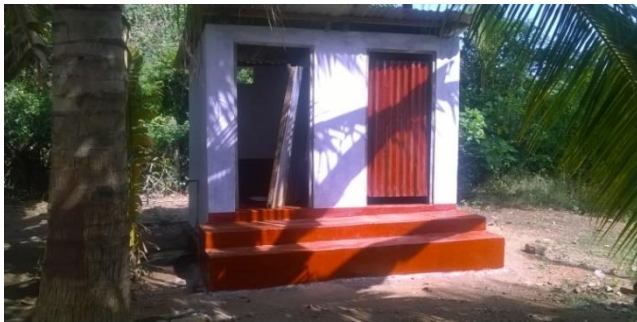
Newly refurbished toilet facilities
