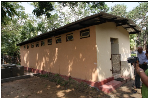
New toilet facilities
