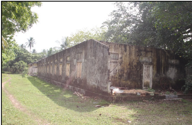
A large dormitory needing total renovation
