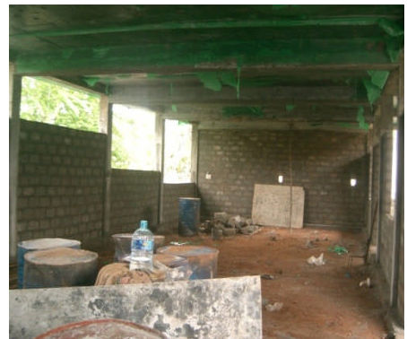
Arobanam Children Home ... a new 3-storey building currently under construction in Mannar
